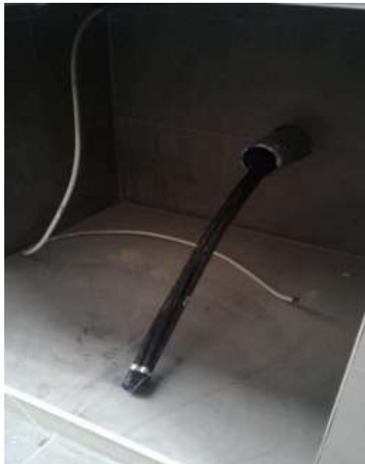
Fig. 13 - Hydraulic hoses in a recess in the diagnostic pit prepared for connection to the hydraulic power supply
