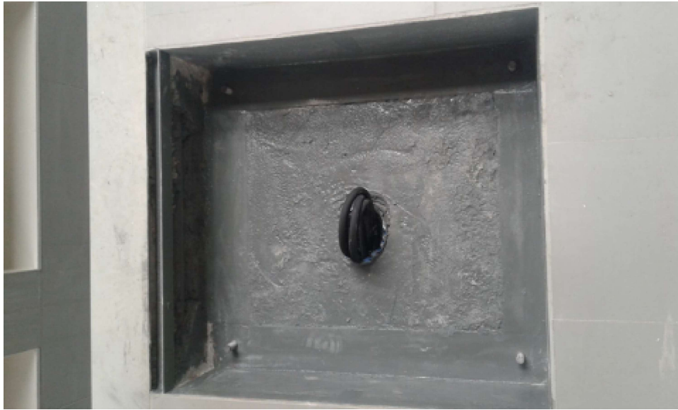
Fig. 12 - View of foundation with hydraulic hoses
