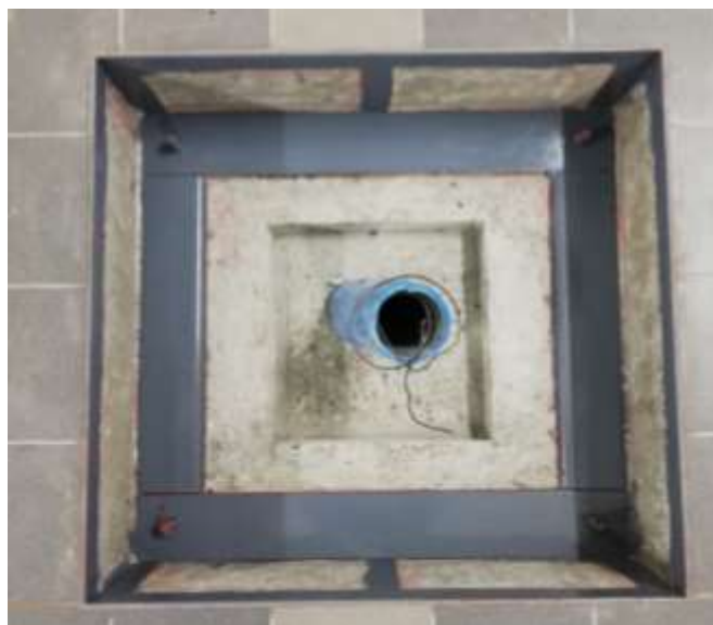
Fig. 9 - SZ-16 foundation and frame
